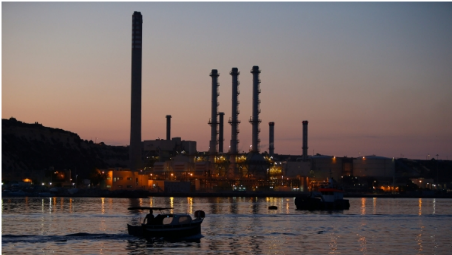
The Delimara site from Marsaxlokk: The old chimney on the left will soon be dismantled.
