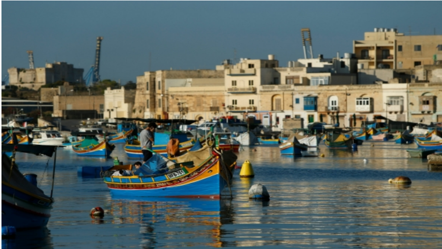
The Delimara power plant site is located on the bay of Marsaxlokk.
